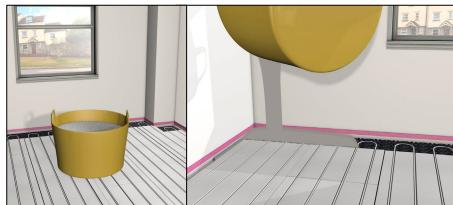
Once sufficient compound has been applied it can be distributed to the required depth using a smoothing trowel or smoothing rake. The surface finish can be improved using a spiked roller.
