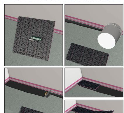
Continue this process to form an entire row of cut-to-size Profix® End-Return Panels running along that end of the room, cutting the final panel to length if required.
