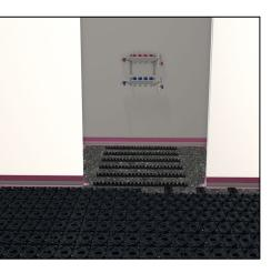
Connect the first pipe run to the manifold.
