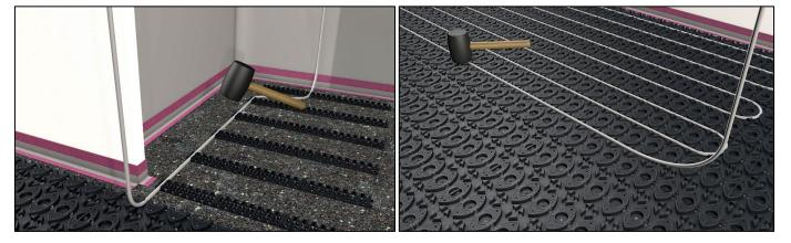
Return the first pipe run to the manifold.
