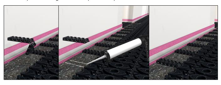
Profix<sup>®</sup> Clip-Rails can also be used in close proximity to the manifold to secure pipework at close centres prior to transitioning into the Profix<sup>®</sup> Panels themselves.
