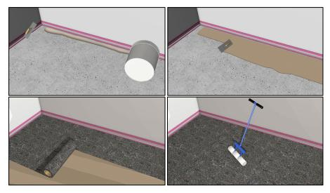
Smooth out the surface of the mats using a roller, pressing down firmly to ensure good adhesion and to remove any air bubbles. Foot traffic should be avoided for 24 hours, while the adhesive dries, before installing the Profix<sup>®</sup> Panels onto the acoustic isolation mats.
