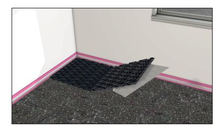
Stick down the panels as before to complete the first row, cutting the final panel in the row to size if required.
