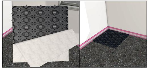
Place the second Profix<sup>®</sup> Panel with the arrow heads facing to the left and engage them into the gates along the right hand edge of the first panel. Peel off the backing sheet on the second panel to expose the adhesive and stick it down.
